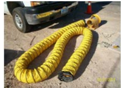
Adequate fresh air blower and vents
